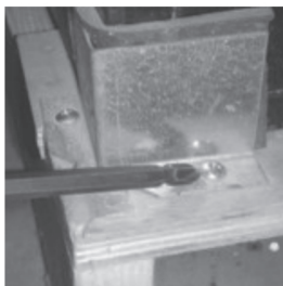
Image 1 Removing bracket from skid
