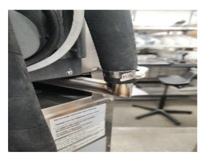
The Hood uses water its filtration system. We recommend having a water line and a drain for this. The amount of water varies on what is being cooked in the oven and at what temperature. The water will be activated ones the hood reaches its temperature threshold parameter.
